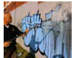
Rinsing larger graffiti after applying BBSM
