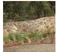
Once clean, re-apply WBGC.
